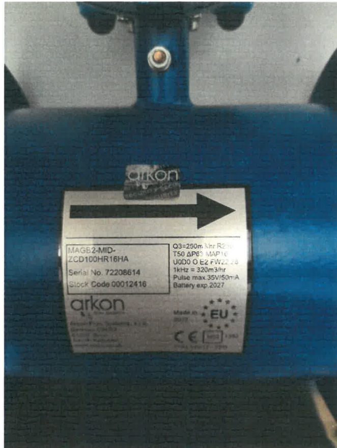
Figure 4: The water meter type MAGB2 – outputs:
